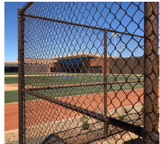
Natina reactive color treatment on the chain-link and poles.
