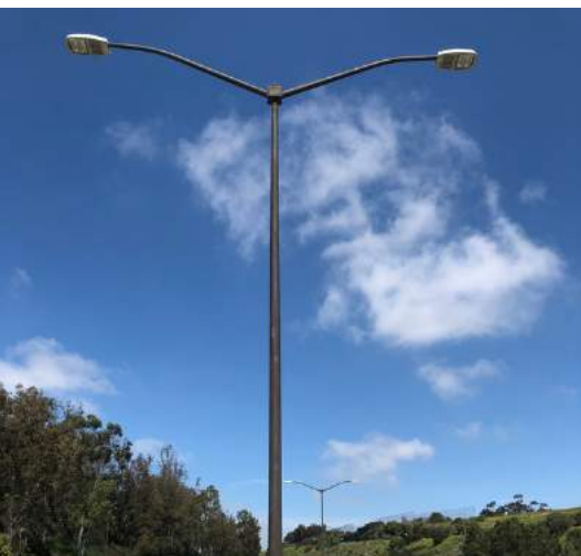
Natina finish on light poles along Florida Drive.
