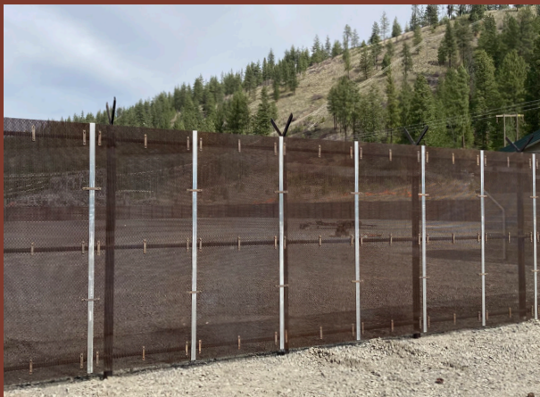
Natina-treated fence around substation.
